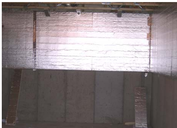
Figure 38. Foil-faced polyisocyanurate insulation
