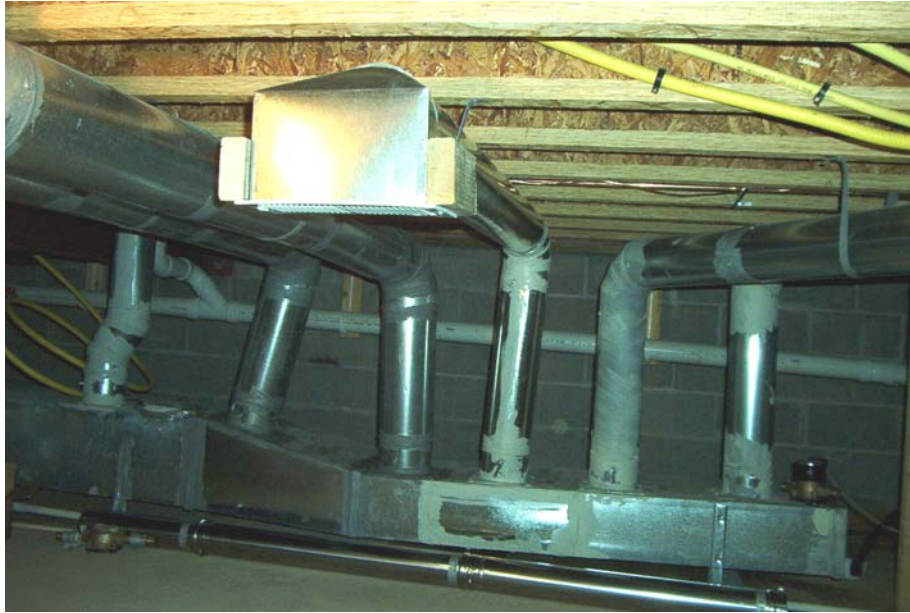
Figure 45. Once the HVAC subcontractor recognized the need to condition the crawl space, a register in the main trunk line was put in. This register was sealed up because it had the potential to divert too much air to the crawl space and a ducted register was installed in a more central location in the crawl space.
