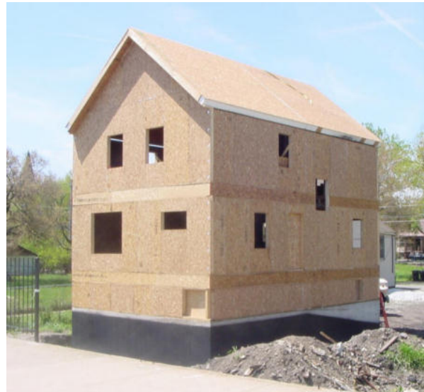
Figure 42. SIPs installed in the first home
