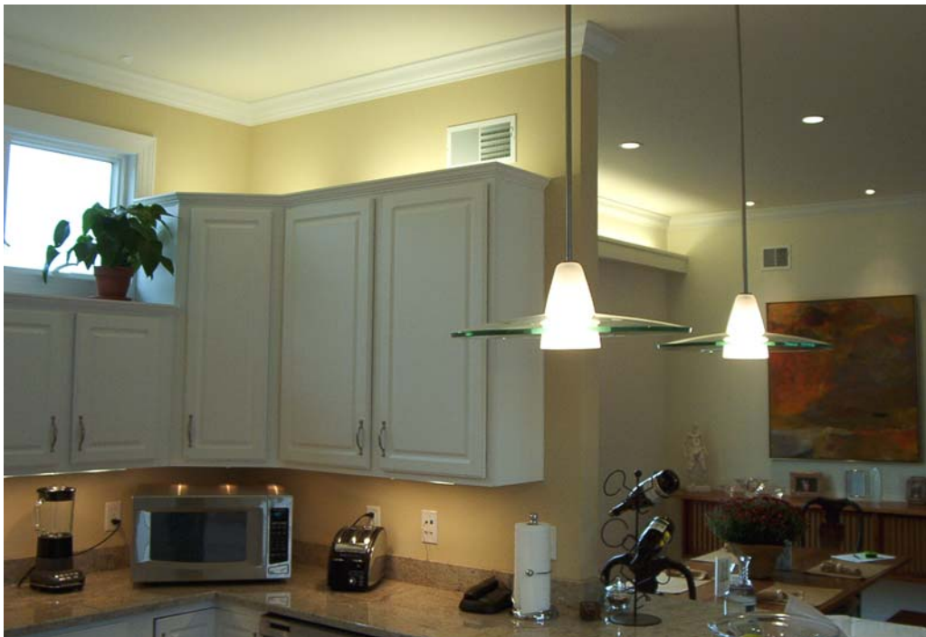
Figure 46. Over-cabinet (fluorescent) and under-cabinet (halogen) lighting was used at the Kacin Construction project. Cove lighting, consisting of strip fluorescent lamps and recessed downlights with CFLs were used in the adjacent dining room.
