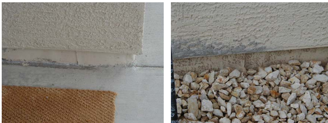
Figure 32. Edge insulation properly protected with sheet metal
