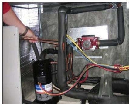
**Figure 3:** Service-friendly heat pump package (left). Classroom unit with room for service (right).
