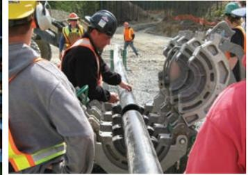
ABOVE DESS HDPE pipe being thermally welded.
