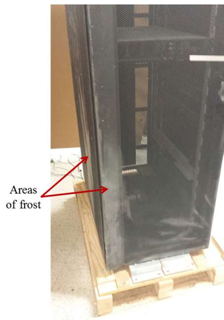
Figure 1 Frost on the covers of an IT equipment rack (also known as a cabinet or frame).
