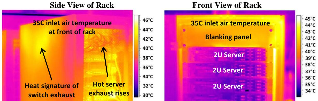
Note how you can see the heat signature of the switch exhaust on the side panel of the rack. Note also how hot the server exhaust is and how it tends to rise to the top of the rack. In the front view of the rack, the blanking panel glows orange indicating how much heat is being trapped behind it.
