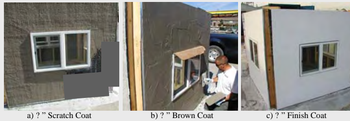
Three-Coat Stucco Wall Assembly
