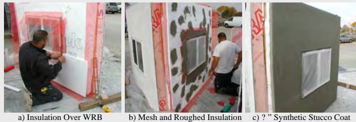
Exterior Insulation Finish System (EIFS) Wall Assembly
