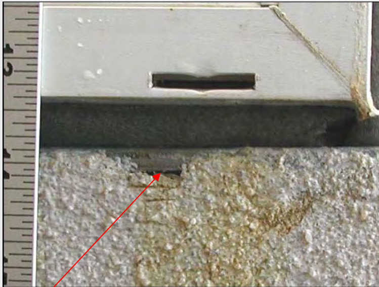
Stucco Flaw Beneath Window Frame
