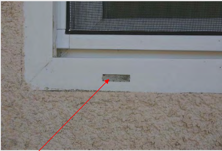
Weep Hole Plugged with Stucco in New Home
