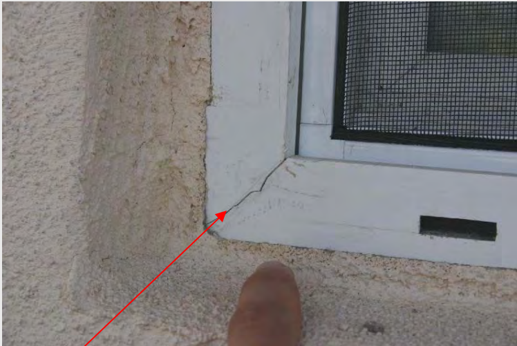
Cracked Window Frame in New Home
