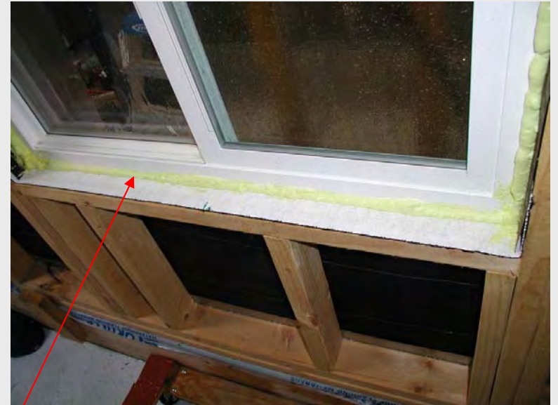
Foam Sealant Contained Leak in This Case
