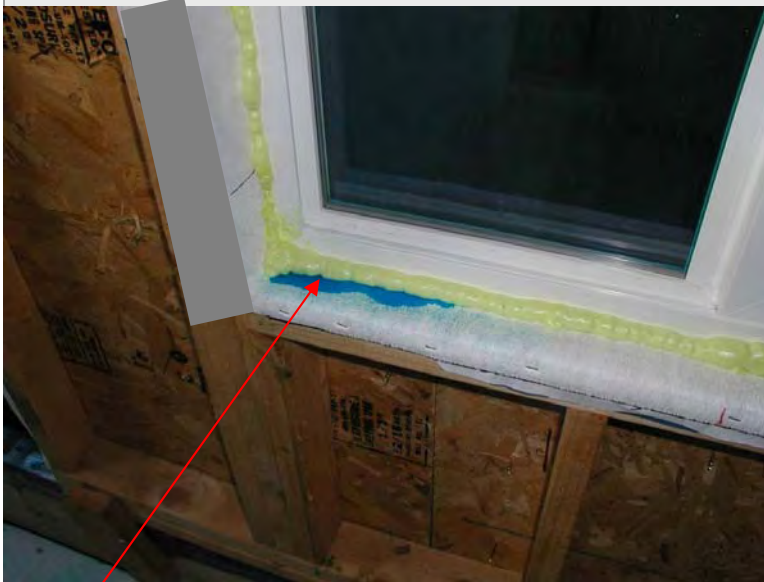
Foam Sealant Did Not Contain Leak in This Case
