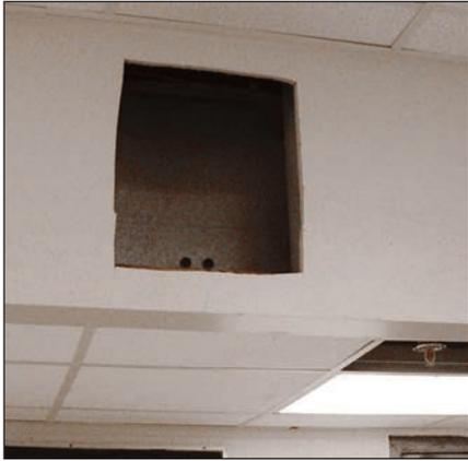
**Figure 5:** A solution for lack of service access to problematic fan motor.
