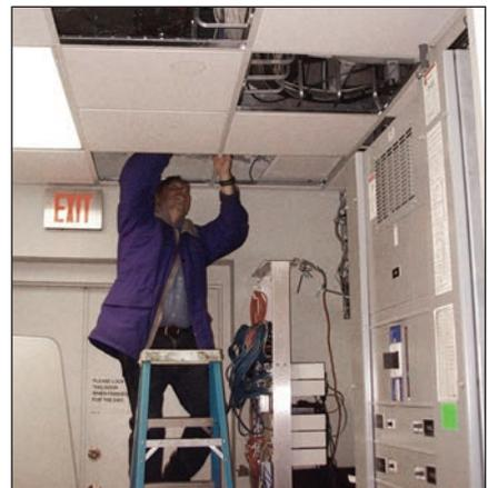
**Figure 4:** Control circuits for "advanced" heat pump. Unit in difficult-to-service location.
