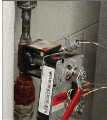
**Figure 8:** Reduced line size control valve caused flow problems.
