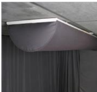
Figure 9.7: Dual Rail system to support half circle or quarter circle fabric ducts
