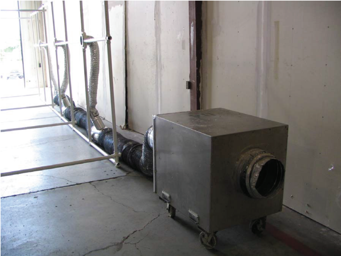
Figure A.4.3 View of the rear wall exhaust ports, 6-inch dampers and branch ducts, 12-inch main duct, and neg-air exhauster.
