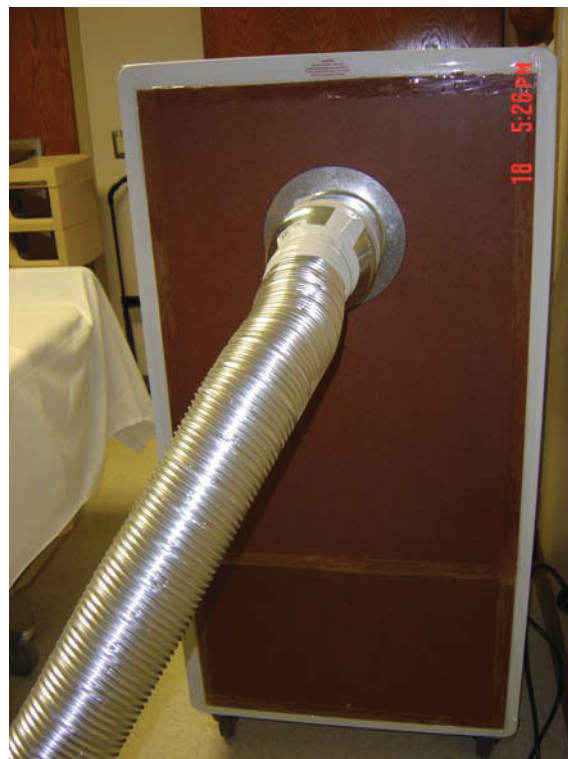
Figure A.2.2 HEPA inlet side adapter for connection to the ventilated headboard exhaust duct.
