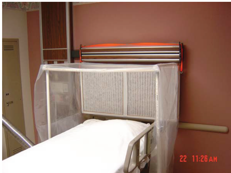
Figure A.2.4 Ventilated headboard with expedient partial patient enclosure in place. The flexible metal hose at left leads to the HEPA filter unit. The frame was constructed from \frac{3}{4} -inch PVC tubing and fittings; 1-inch tubing and fittings would provide a more rigid frame.
