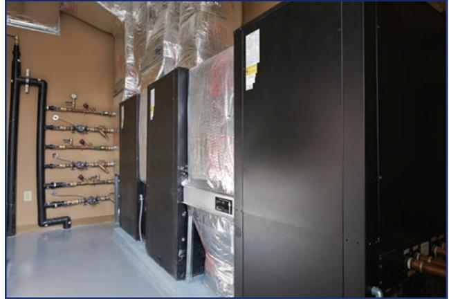
**PHOTO 4** Easy to access heat pumps and one common filter size makes operation and maintenance easier.
