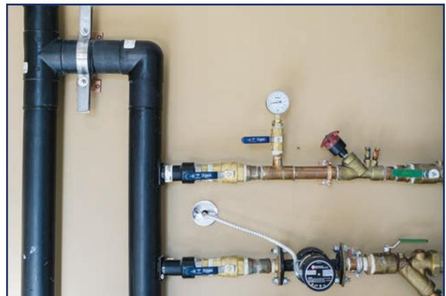
PHOTO 2 Single pipe loop system. Heat pumps are supplied and returned from a common pipe.
