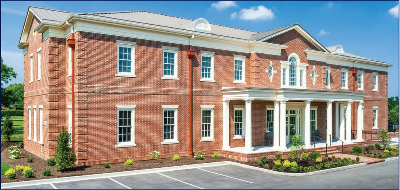
PHOTO 1 The newly constructed two-story, 11,750 ft<sup>2</sup> (1092 m<sup>2</sup>) CMTA Lexington Office in Lexington, Ky. Using insulated concrete form (ICF) construction provided a high resistivity to heat flow with a value of R-40.
