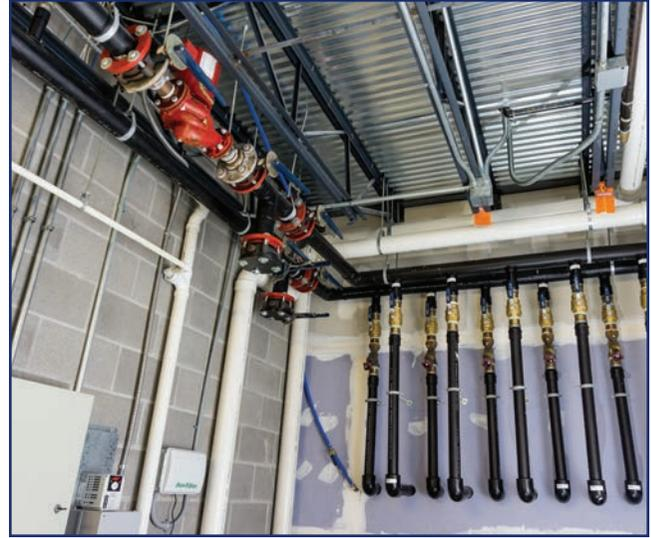
**PHOTO 3** Geothermal entrance and centralized variable speed loop pump. Easy access to well field isolation.
